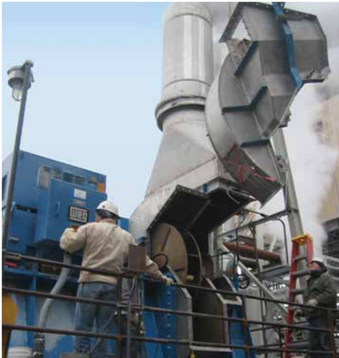
FD FAN - MINERAL SALTS - USA DRBS 1700 SR. 53 SWSI, Radial Bladed Draft Fan, Arrangement 7B Performance: 63,000 cfm, 67.0 in wg SP, Den. 0.0638 lb/ft 3 , 1785 rpm and 901 BHP
